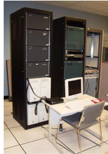
Internet Lab at UVA. with Cisco 7010 routers
